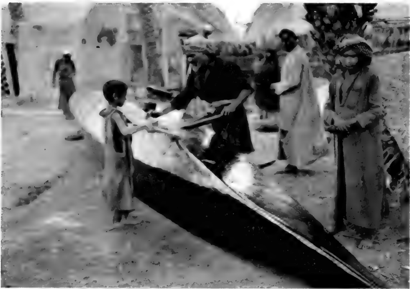
Fig. 2. Tarring the skin used to cover the framework of the boat
